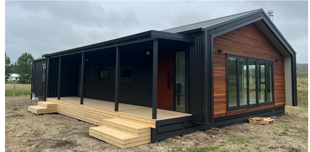
Elsthorpe 139m 2 | 4 bedrooms | 2 bathrooms | 1 office
